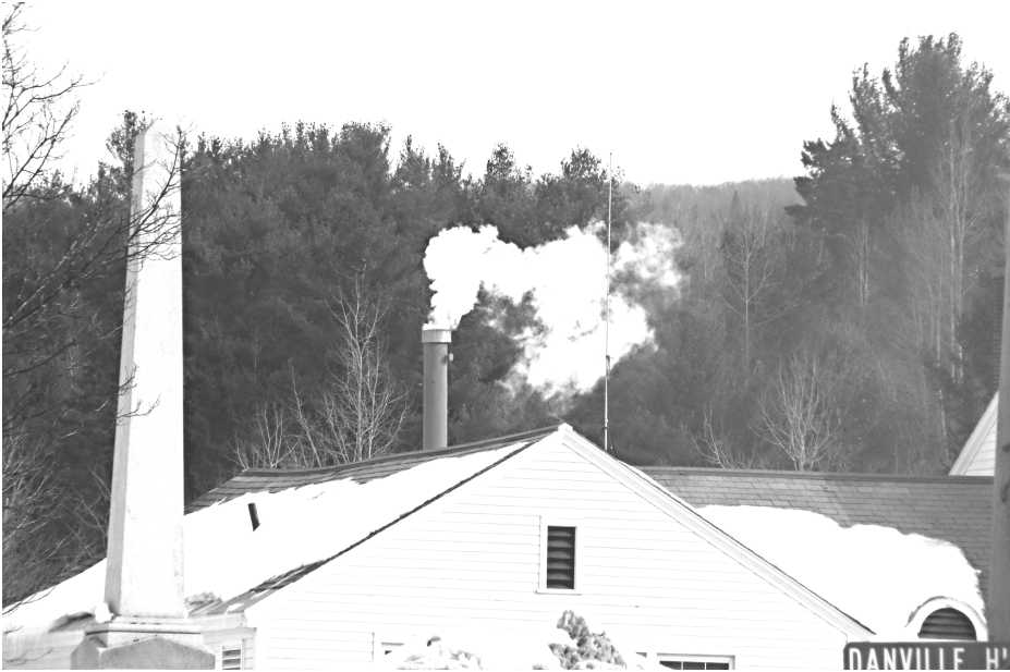
Smoke can be seen rising from the school's woodburning heating plant. The plant has gone through a few test burns and is now being used regularly. Cabot School Board Chair Chris Tormey said that wood chips should cost half the price of oil and will replace 80 percent of the oil used. Photo courtesy of Will Walters.
