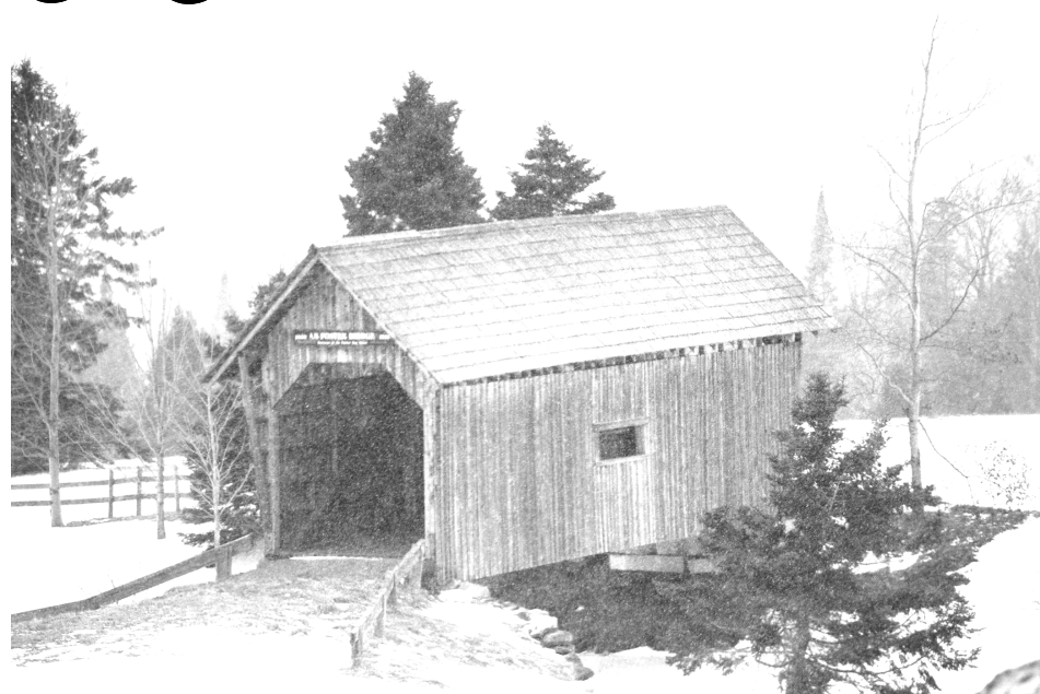
Cabot Plains Bridge - Photo Courtesy of Anne Nadel
