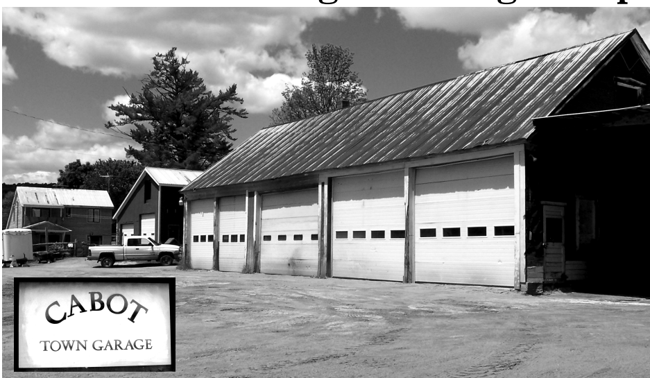
Cabot Town Garage in Cabot Village.
