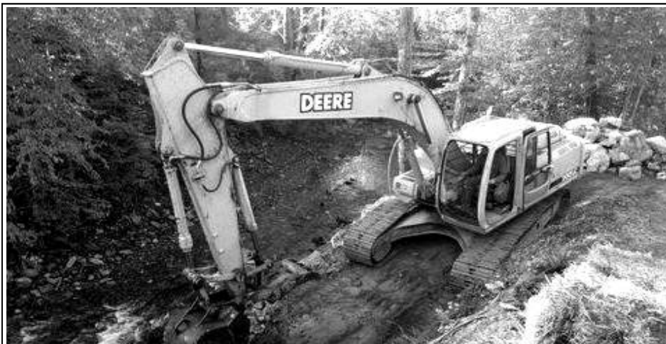
Lajeunesse Construction began work on the Cabot Town Garage August 17. Since the contract was signed, tons and tons of earth have been moved and the project is beginning to take shape. Photo by Brad Alexander.
