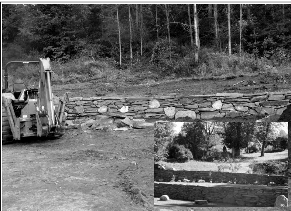
A rock wall behind the Wiley Building is being constructed by Richard Ducharme of Cabot, to enhance and shape the new parking area. Another completed project by Mr. Ducharme is on the Westervelt property (inset).
