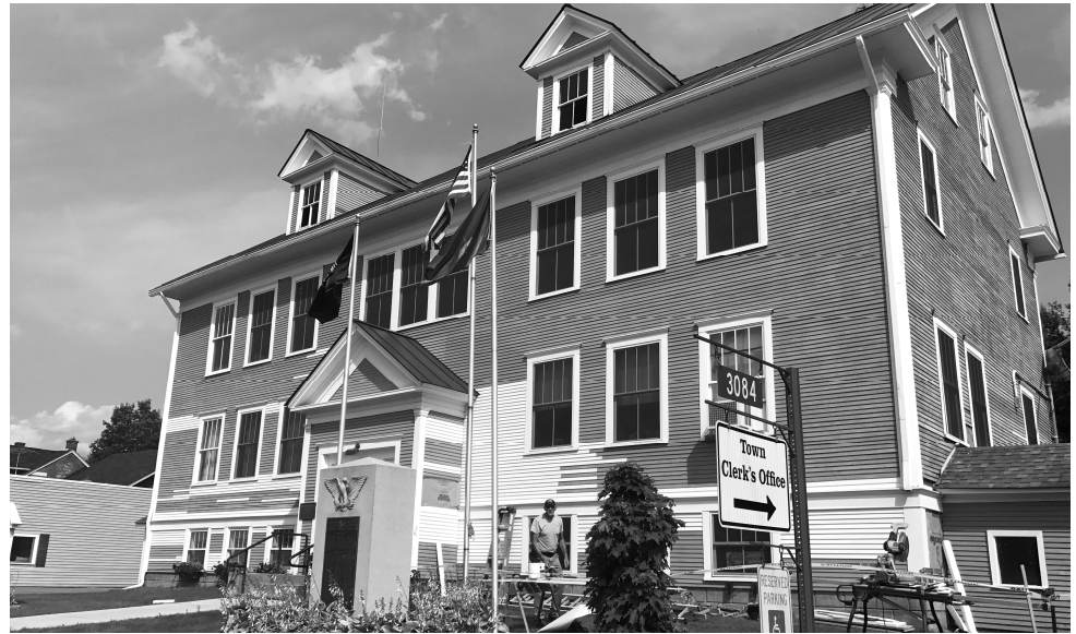
George Colgrove is replacing siding before the Wiley Building is painted. Jeanne Johnson photo.
