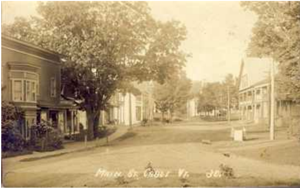
Note: A century-old picture postcard shows the northeast section of the Voodry building, now 3065 Main Street, with gas pumps in front of Harry's Hardware in the background.
