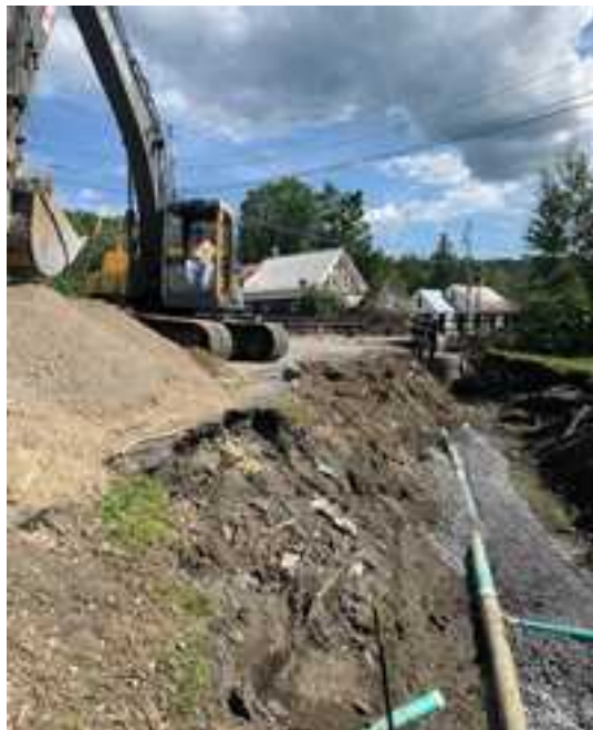
Cabot bridge work at intersection of 215 N and S Walden Road.
