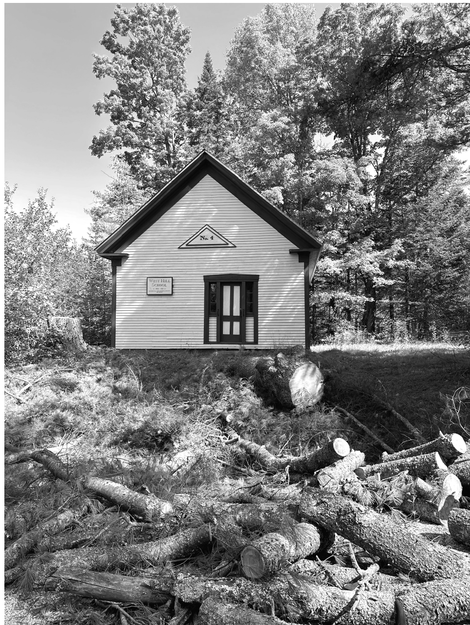
Hazardous Tree Being Removed at Old School House.
