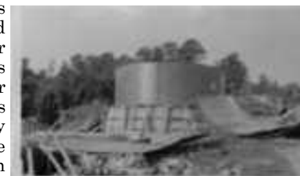
The surge tank under construction. It was perched on top of the hill high above the power plant. Heavy steel pipe carried water down the steep hillside from the surge tank to the power plant located on the Winooski River, not far from Route 215S and the Cabot/Marshfield town line. Photo by John C. Donahue, electrical engineer, courtesy of Cabot Historical Society.
