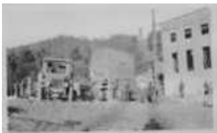
Construction of the power plant near what is now U.S. Route 215S. Photo by John C. Donahue, electrical engineer, courtesy of Cabot Historical Society.
