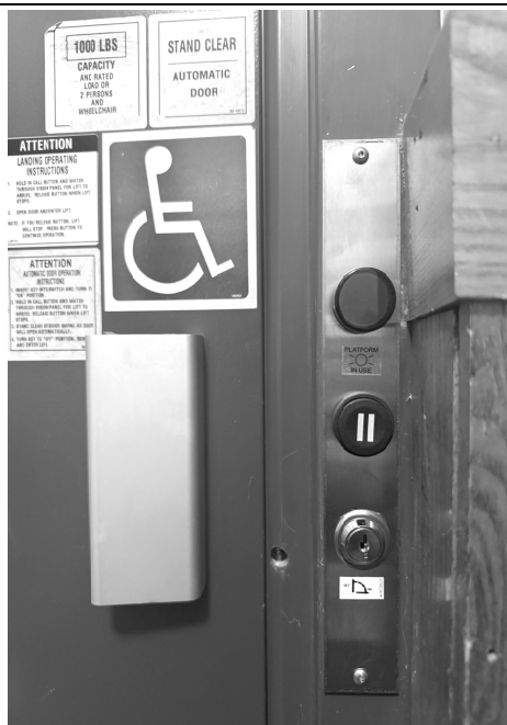
New lift call button pad—turn the key and push the button.
